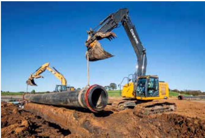
Pipes go in at Ravenswood in Menlo Park (Ivan Parr)
