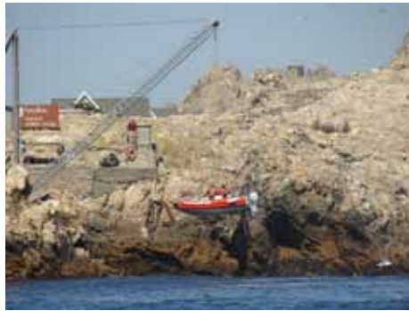
East Landing crane on Southeast Farallon Island
