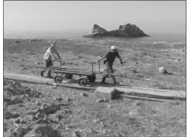
Volunteers Jeb Boba (left) and Dave Stalthers used Farallon Railways to move the pipe in preparation for removal.
