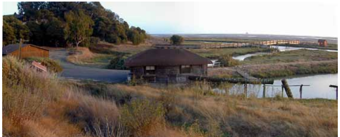
Pump house that had been renovated into an environmental education classroom. Photo by Dr. Chris Kitting
