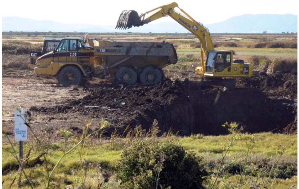
Restoration at Cullinan Ranch. Photo: Don Brubaker
