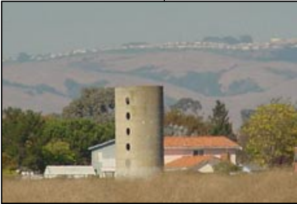
Silo in Mayhew's Landing. Photo: Katie Fotta, USFWS
